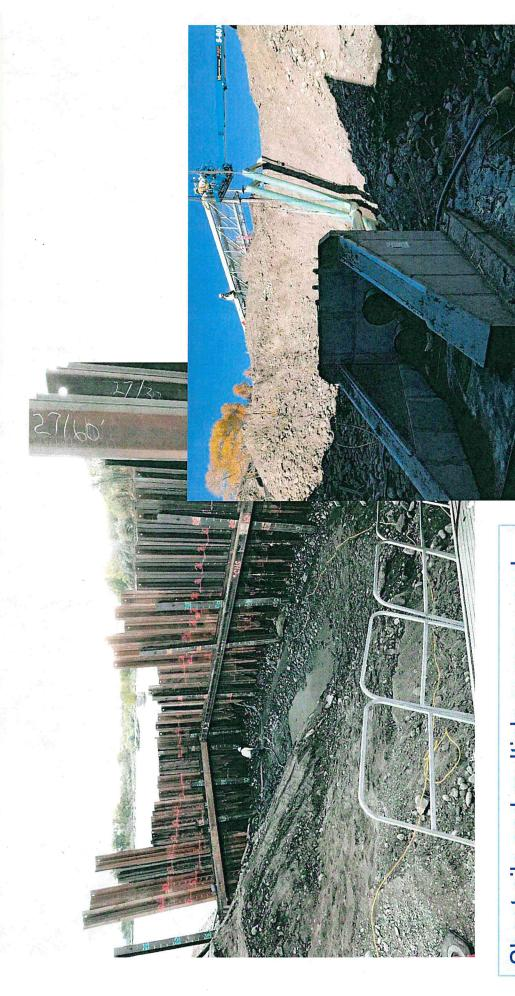
Sheet pile and multiple pumps used to allow the diffuser to be safely and securely installed on the river bottom.
