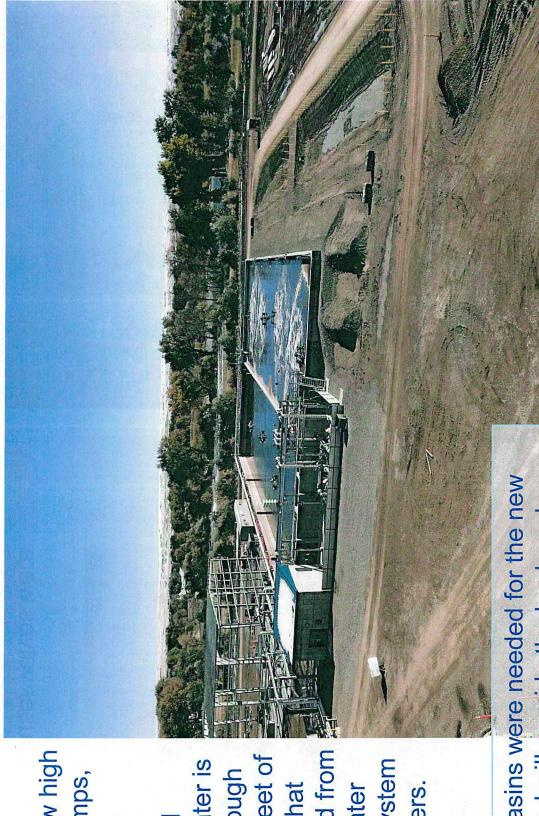
The new basins were needed for the new diffusers and will provide the backwash water for the new arsenic multimedia filters.
