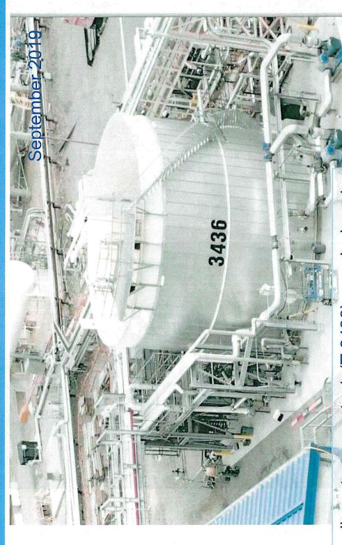
A new oily water surge tank (T-3436) was designed, purpose is to improve oil & grease removal on the constructed and is now in operation. Primary front end of the treatment system.
